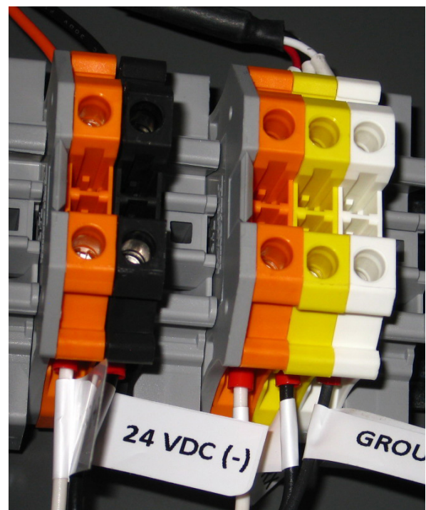
Figure 14. Wire Termination
